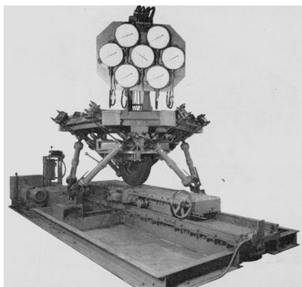
(a) Tyre test machine proposed by Gough [55]
